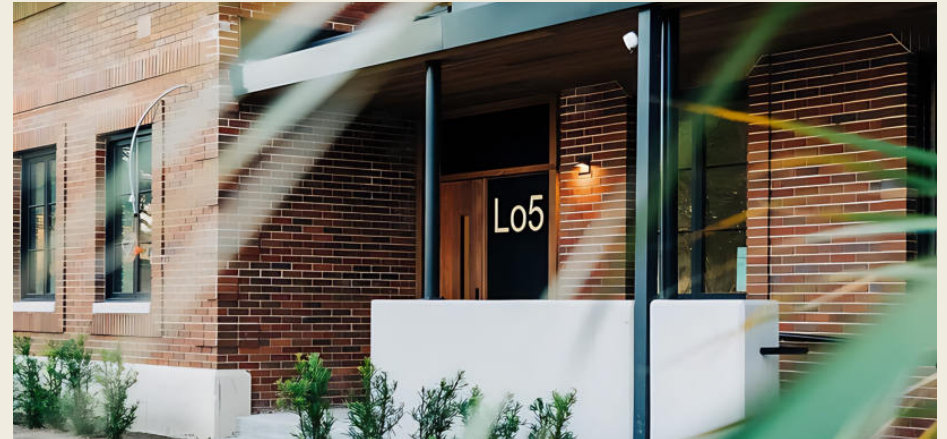
FIG. 04 Porch entry at the Fifth Street elevation.
